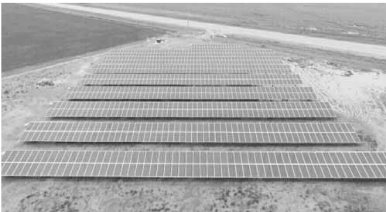
The Cotton Electric Cooperative Community Solar project, owned by WFEC, consists of 950 solar modules each rated at 315 Watts. The entire site is rated for 250 kilowatt hours (kWh) at peak performance.
