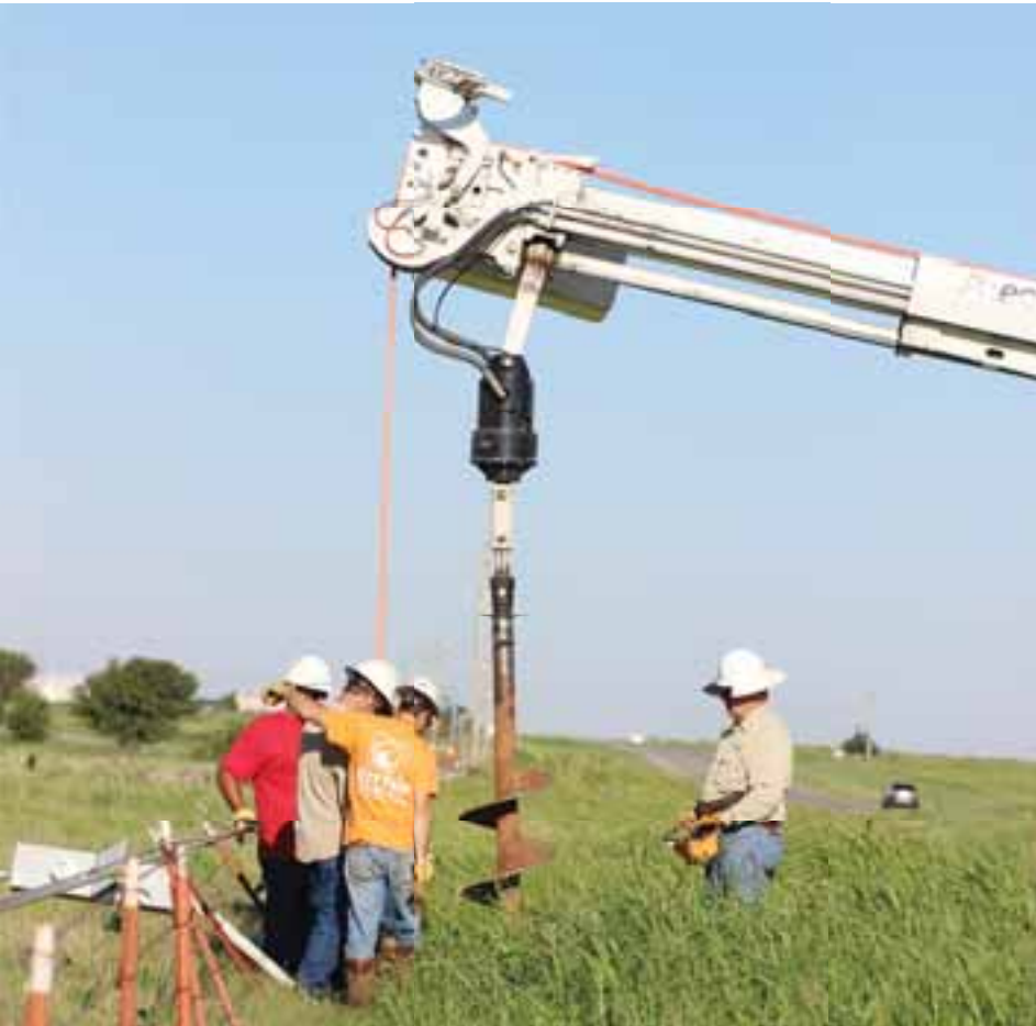
Once a damaged pole is extracted, a new hole is dug into the ground to make room for a replacement pole. From left, Journeyman Linemen Shayne White and Kyle Linthicum join Ledford and Ballard to prepare for a new utility pole.
