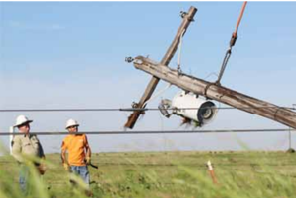
Heavy Equipment Operator Chuck Ballard, left, remotely operates a bucket truck to lift a broken utility pole out of the ground with the assistance of Vegetation Management Worker Ryan Ledford. The pole was damaged during the July 30 storm.
