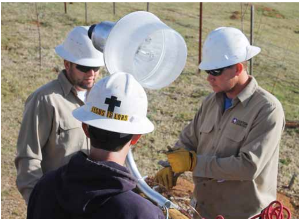
Apprentice linemen Jeremy Crabtree, left, and Seth Walters, right, attach a light to a pole while journeyman lineman Tyson Potter observes.
