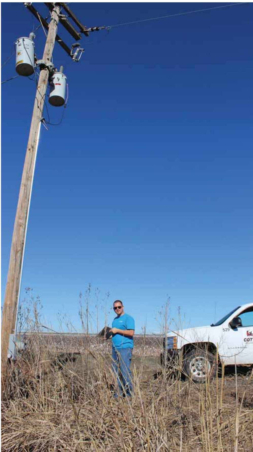
Many of the meters Josh Belcher visits each month are in out-of-the-way spots. He drives through a cotton patch to reach this one located along a fence line. See story, Page 8.
