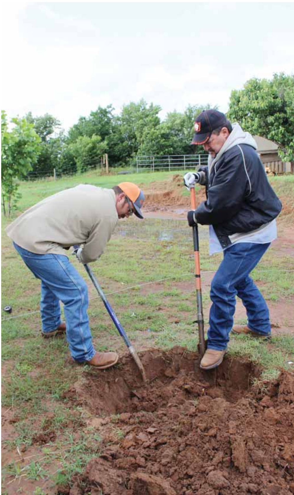
The wettest May on record meant journeyman lineman Chad Cowan, left, and heavy equipment operator Darrell Loveday spent a lot of time with shovels. The trencher Loveday normally uses for large and small digs was too heavy for the saturated ground. This meant all new services requiring long trenches were postponed until the ground dried and the trencher could be used without leaving huge ruts along the work path.
