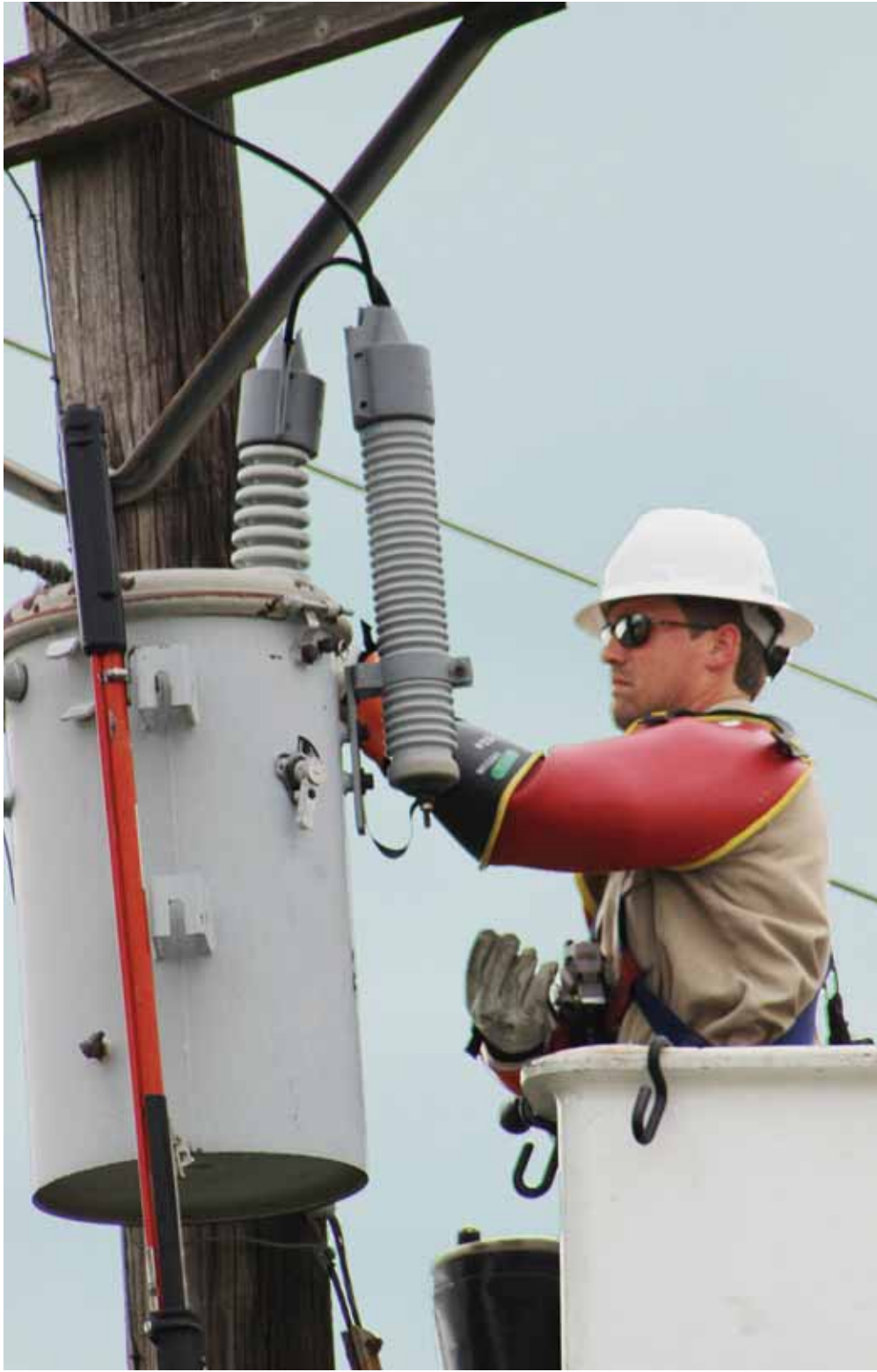
This shot of Matt Winburn working on a transformer shows some of the safety equipment Shelly Sehrt tests (see story, Page 11). The long orange pole is called a hot stick. The insulated device extends a lineman's reach. The elbow-length rubber gloves are Class 3, indicated by the green label. They should withstand up to 30,000 volts. Leather protectors go over the rubber gloves to prevent punctures. Rubber sleeves extend from Winburn's shoulders and tuck into the rubber gloves. While not tested, a hard hat, safety glasses and a fire-retardant long-sleeved shirt also protect the lineman. A blue harness tethers him to the insulated bucket as a fall-restraint.
