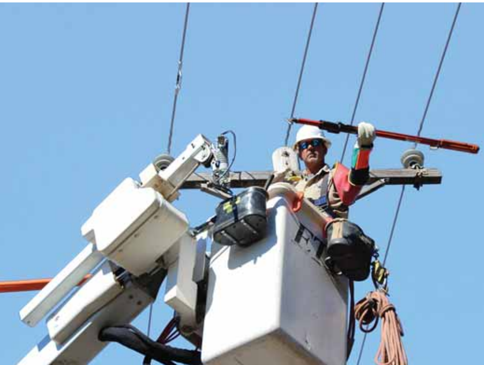
Linemen wear personal protection equipment (PPE) from head to toe to keep them safe. Everything Jarrod Hooper is wearing is an article of PPE: Hard hat, sunglasses, 100 percent cotton long-sleeve shirt treated with fire retardant, safety harness, rubber sleeves, high-voltage rubber gloves and leather glove protectors. He is wearing jeans also treated with a fire retardant and steel-toed boots. The truck is grounded and the bucket is insulated, as are the bright orange hot stick and line hose.
