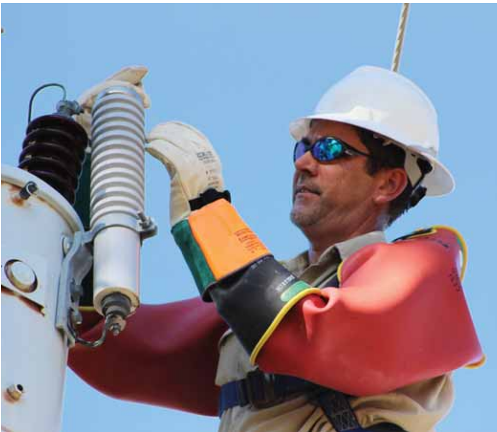
Linemen wear personal protection equipment (PPE) from head to toe to keep them safe. Everything Jarrod Hooper is wearing is an article of PPE: Hard hat, sunglasses, 100 percent cotton long-sleeve shirt treated with fire retardant, safety harness, rubber sleeves, high-voltage rubber gloves and leather glove protectors. He is wearing jeans also treated with a fire retardant and steel-toed boots. The truck is grounded and the bucket is insulated, as are the bright orange hot stick and line hose.
