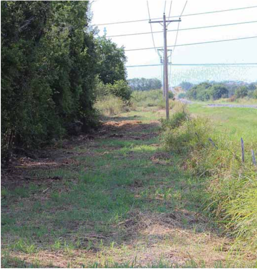
Rapid regrowth of native grasses is seen as a big advantage of new machinery used when clearing Cotton Electric rights-of-way. In the photo above, Johnson grass has sprung up in an area cleared only a few days earlier. The photo below demonstrates the selective nature of herbicides used below power lines to retard new tree growth while allowing grasses to thrive.
