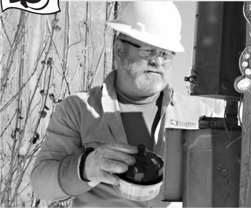
Journeyman field meter technician Rex Hiebert changes a meter on one of his daily stops.
