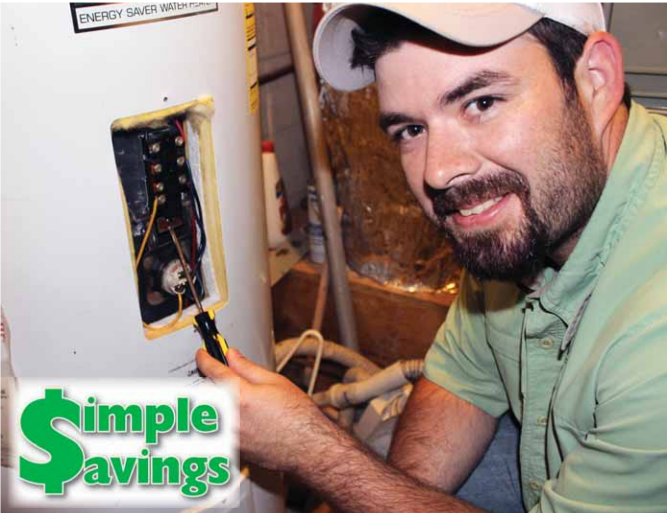
A screwdriver is usually the only tool needed to adjust the thermostat on a water heater. Remember to turn power off at the breaker before working on any electrical appliance.
