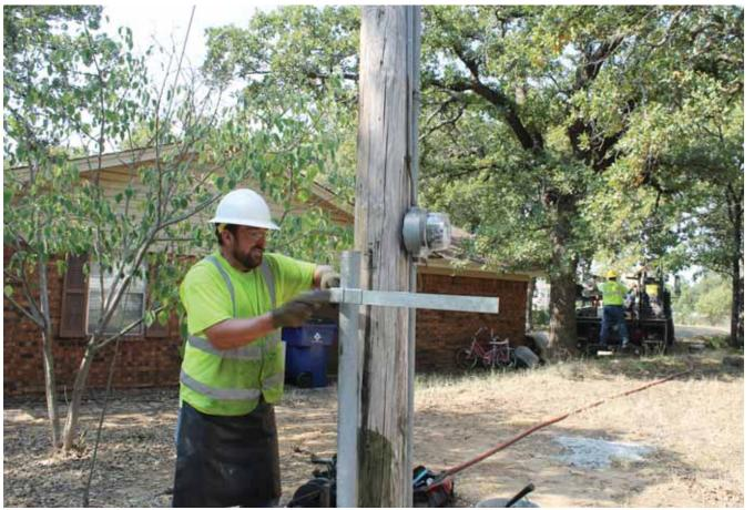
A worker tightly wraps galvanized bands around the pole and truss as part of the restoration.
