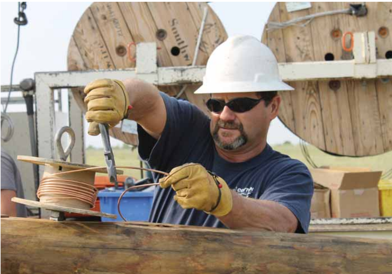
Roy Mason cuts a length of grounding wire to be attached to a power pole.
