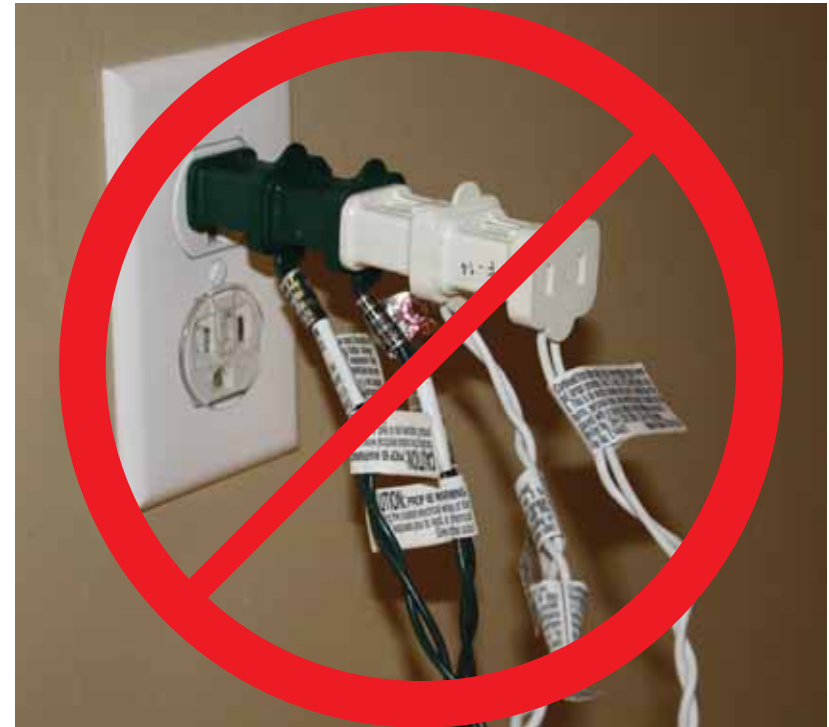
One of the riskiest holiday behaviors is overloading your electrical outlets. Plugging strand after strand of outdoor or tree lights together, plugging them into an extension cord and plugging that into an outlet will overload the outlet. Plugging multiple strands of cords into a power strip does not add any juice to the electrical circuit that powers the outlet you plug the strip into.
