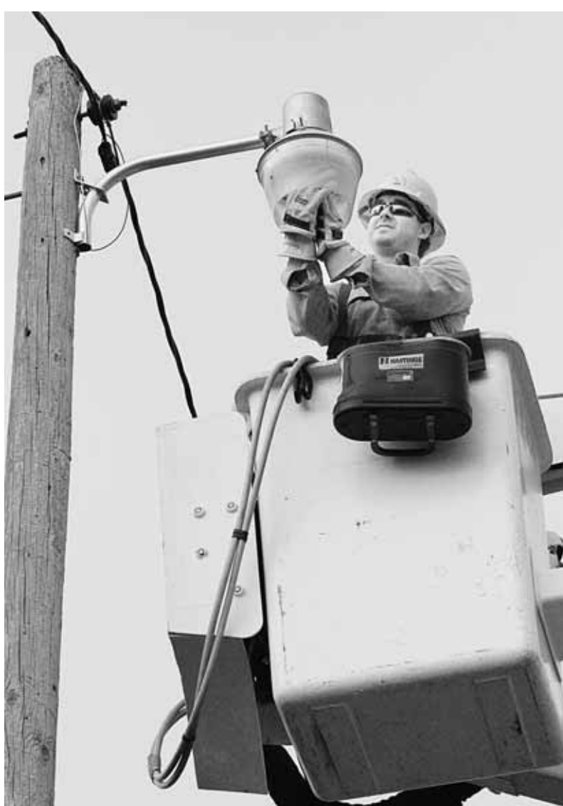
Evan Hays performs maintenance on a security light in the Medicine Park area.
