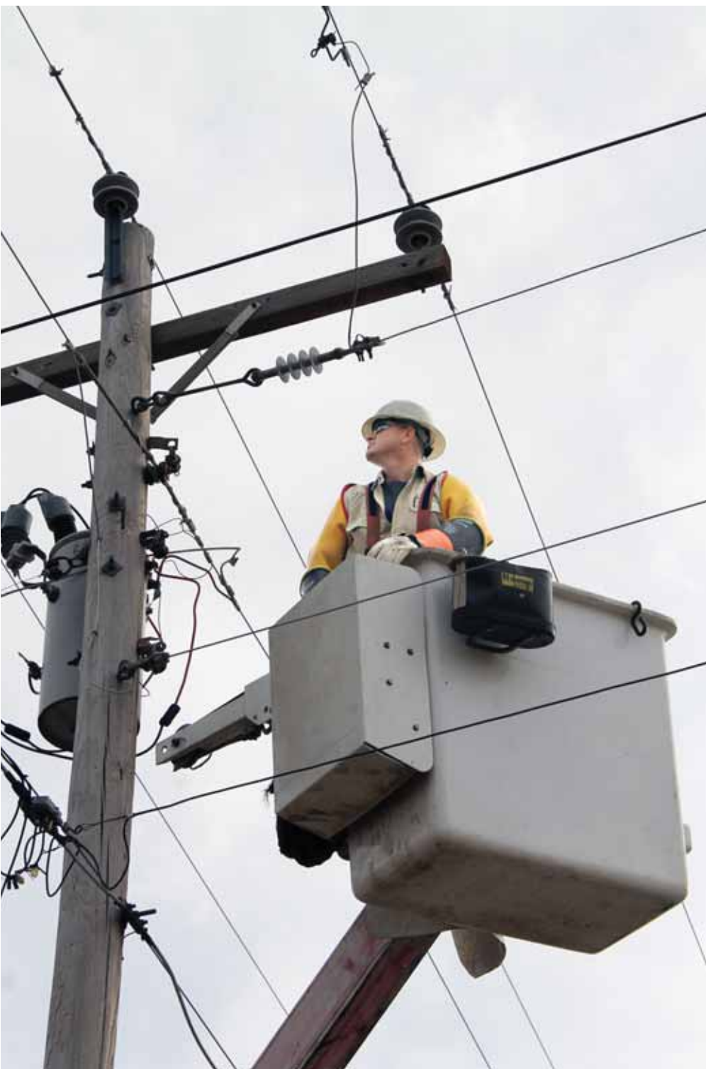
Journeyman lineman Scott Dennis said reworking transformers is one way he and fellow Cotton Electric line workers help improve the quality of power delivered to the co-op’s members.
