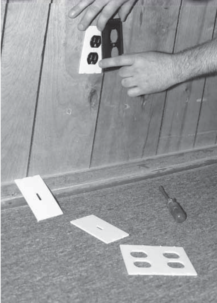
Wall sockets can be sources of air drafts. Pre-cut foam insulation is inexpensive and simple to install.
