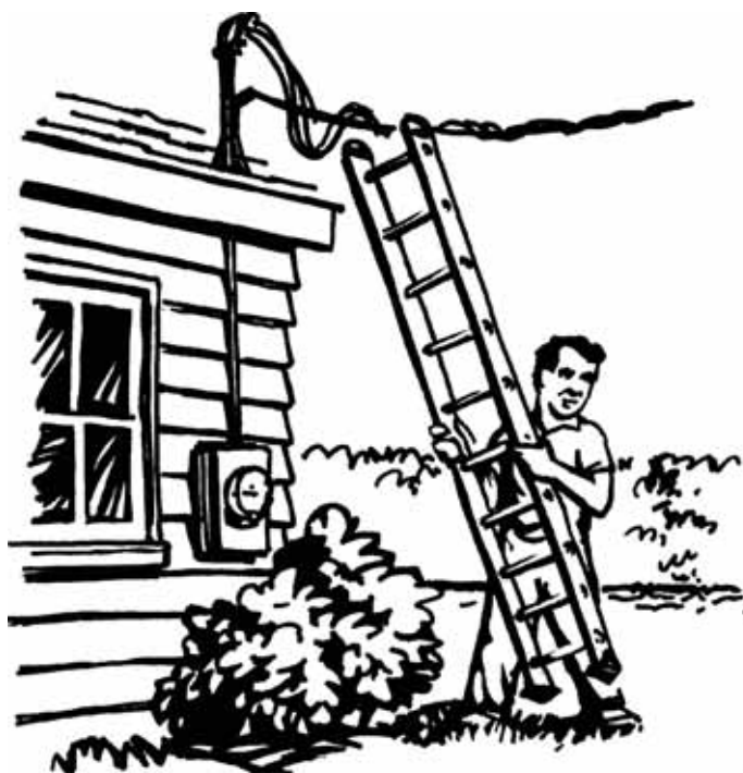
Always look up before positioning a ladder.
