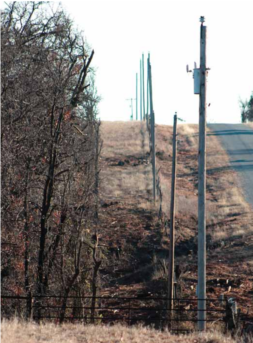
A few days later, the same site has had some trees removed, branches from others trimmed back to a safe distance from the power lines. Crews will revisit over the years with herbicides and to trim again if needed.
