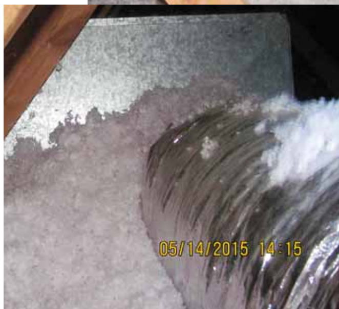
On his return visit a year later, Stephens found the insulation in the attic had been supplemented to a level that would retain conditioned air in the Smith home more efficiently. At left, a new air duct is securely attached to the air handler.
