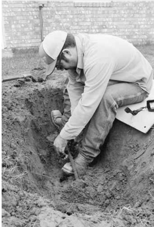
Chad Cowan repairs a faulty segment of underground line.
