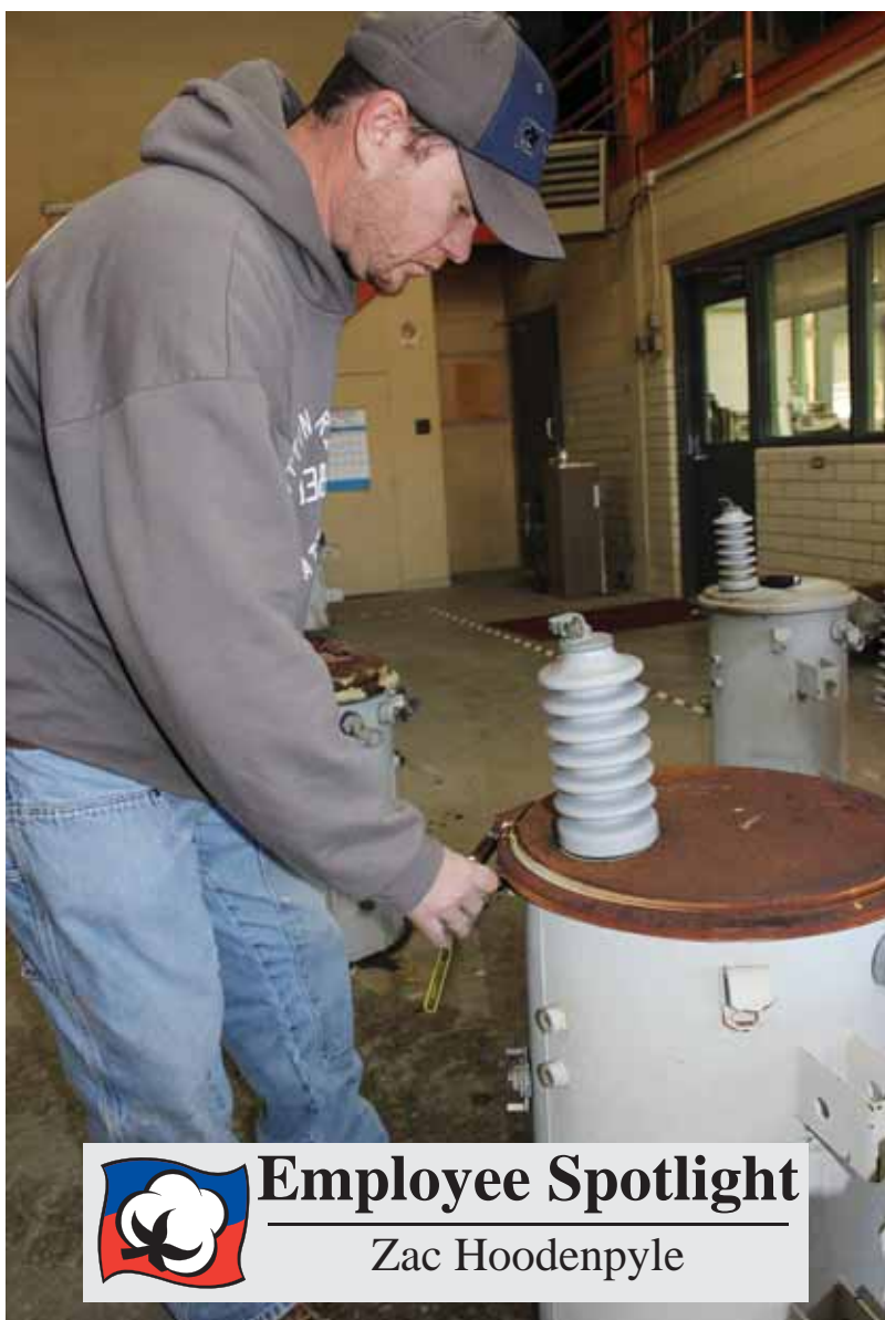
At left, Zac Hoodenpyle begins the refurbishing process by opening up transformers. The parts inside, above, are immersed in a non-conductive oil.
