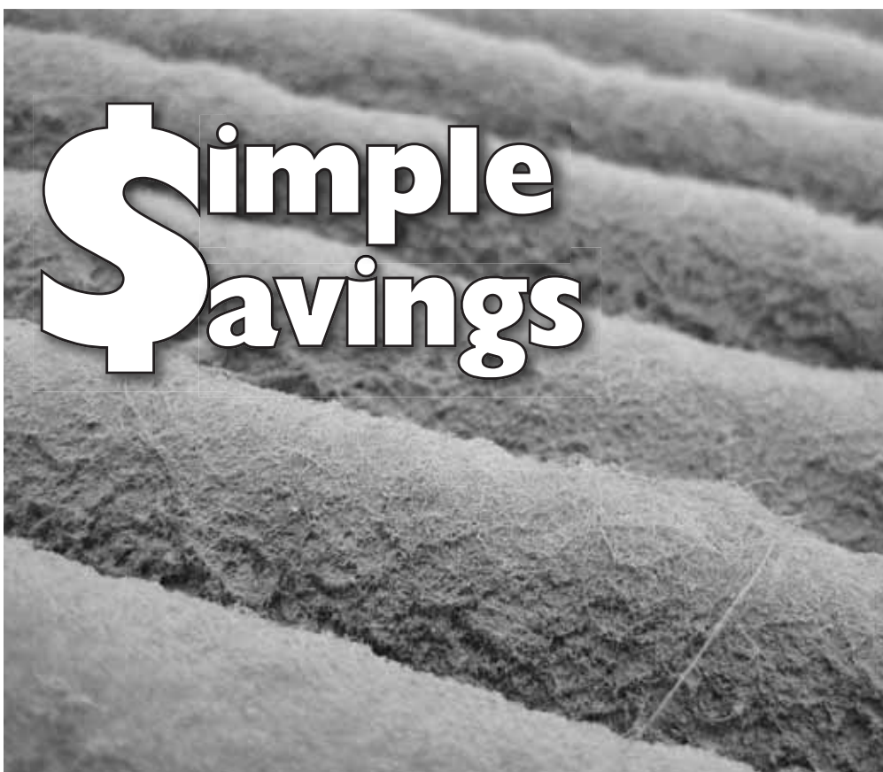
How do you know when a filter must be replaced? Check to see if air can get through. This dirty filter was left in place for six months — layers of dirt and hair prevent air from entering the home's HVAC system.
