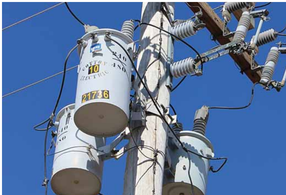
Cotton Electric transformers may be installed as singles or in groups as shown above, depending on the electrical requirements at a location. The yellow 10 indicates the kVA of the unit. The 240/480 indicates voltage, and 21736 is a serial number assigned by the co-op.
