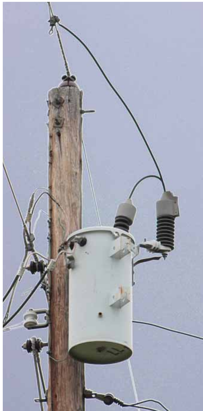
Above, journeyman lineman Matt Winburn begins to rework a transformer. Below, all connections have been tightened and insulated bird wire and bushings installed. This 15-minute bit of maintenance means this transformer is unlikely to be the source of a long outage caused by wildlife.
