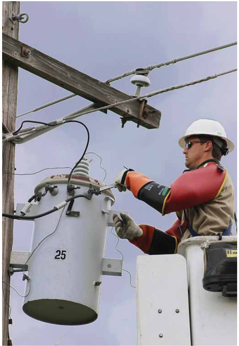
Above, journeyman lineman Matt Winburn begins to rework a transformer. Below, all connections have been tightened and insulated bird wire and bushings installed. This 15-minute bit of maintenance means this transformer is unlikely to be the source of a long outage caused by wildlife.
