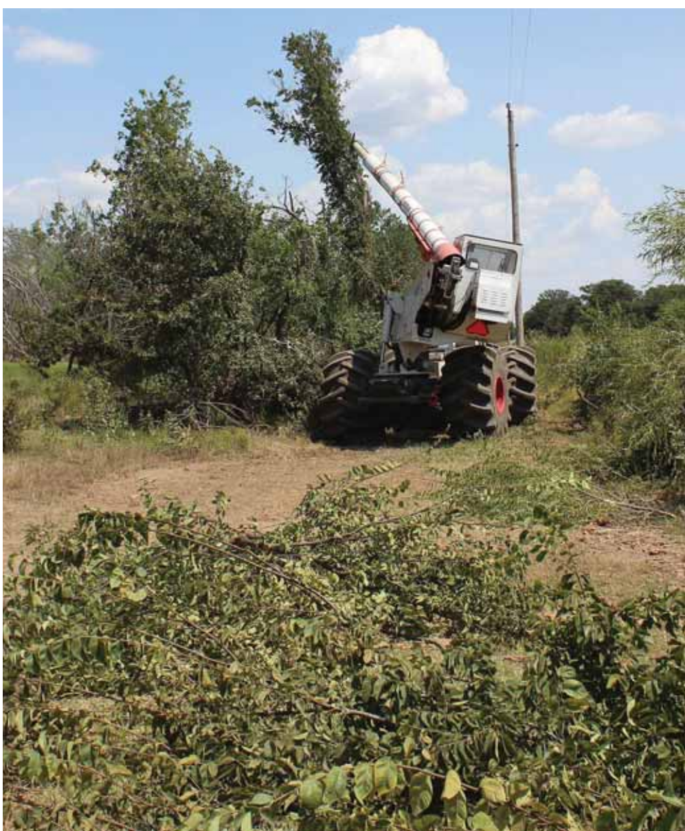
In the top two photos, Cotton Electric's contractor coordinator Mike Darnell visits a site the day before and the day after the NRS right-of-way crew cleared vegetation away from Cotton Electric lines. The bottom two photos show the precision achieved with a Kershaw telescoping tree trimmer. Darnell said the tops of nearby trees are trimmed to taper away from power lines. If the tree falls at some point in the future, it is less likely to damage the lines and could prevent a long-term outage. During the 2010 ice storm, a tree fell and took down a mile of line. It took several days to rebuild. More photos of tree-trimming machinery results are on Pages 12 and 24.
