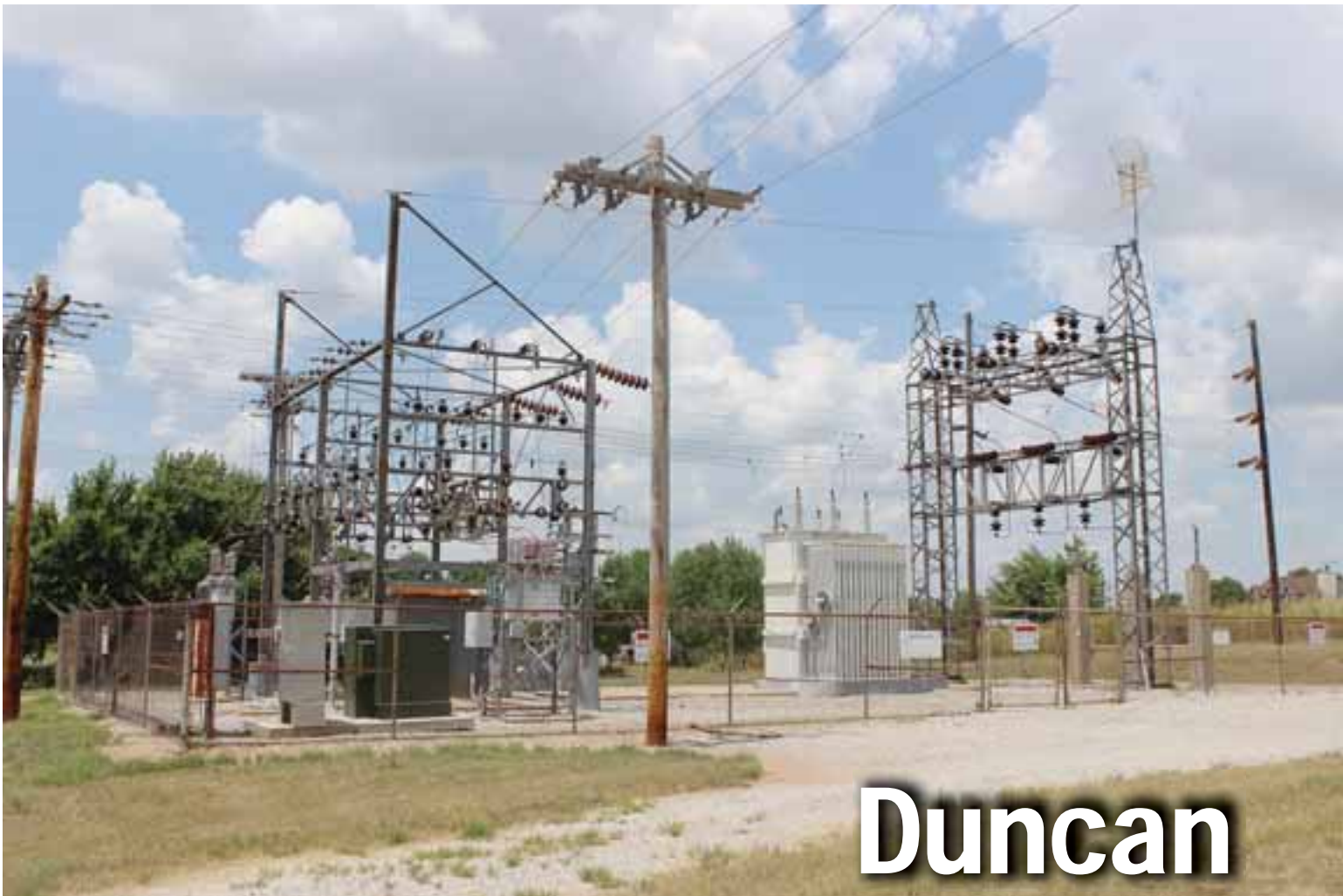
Looking south from the Duncan sub, power leaves substations via 3-phase distribution poles, headed in all directions to serve Cotton Electric members.
