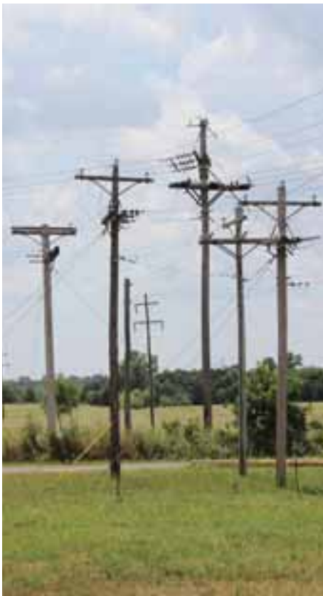
Looking south from the Duncan sub, power leaves substations via 3-phase distribution poles, headed in all directions to serve Cotton Electric members.
