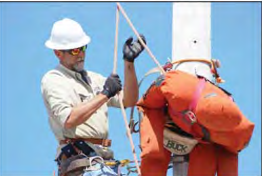
Journeyman Lineman Jarrod Hooper prepares to lower the “hurt man” to safety during pole top rescue.
