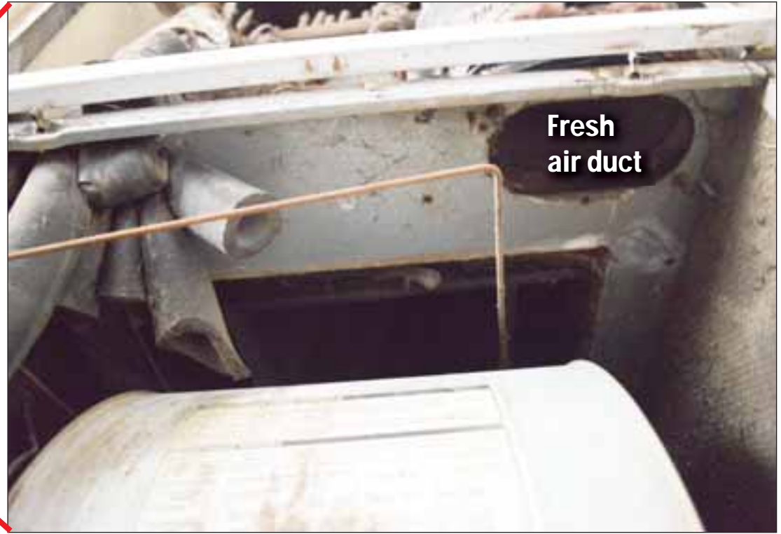
A fresh air duct allows air from outside the house to enter the furnace where it is conditioned by the coil to add air circulation throughout the home.
