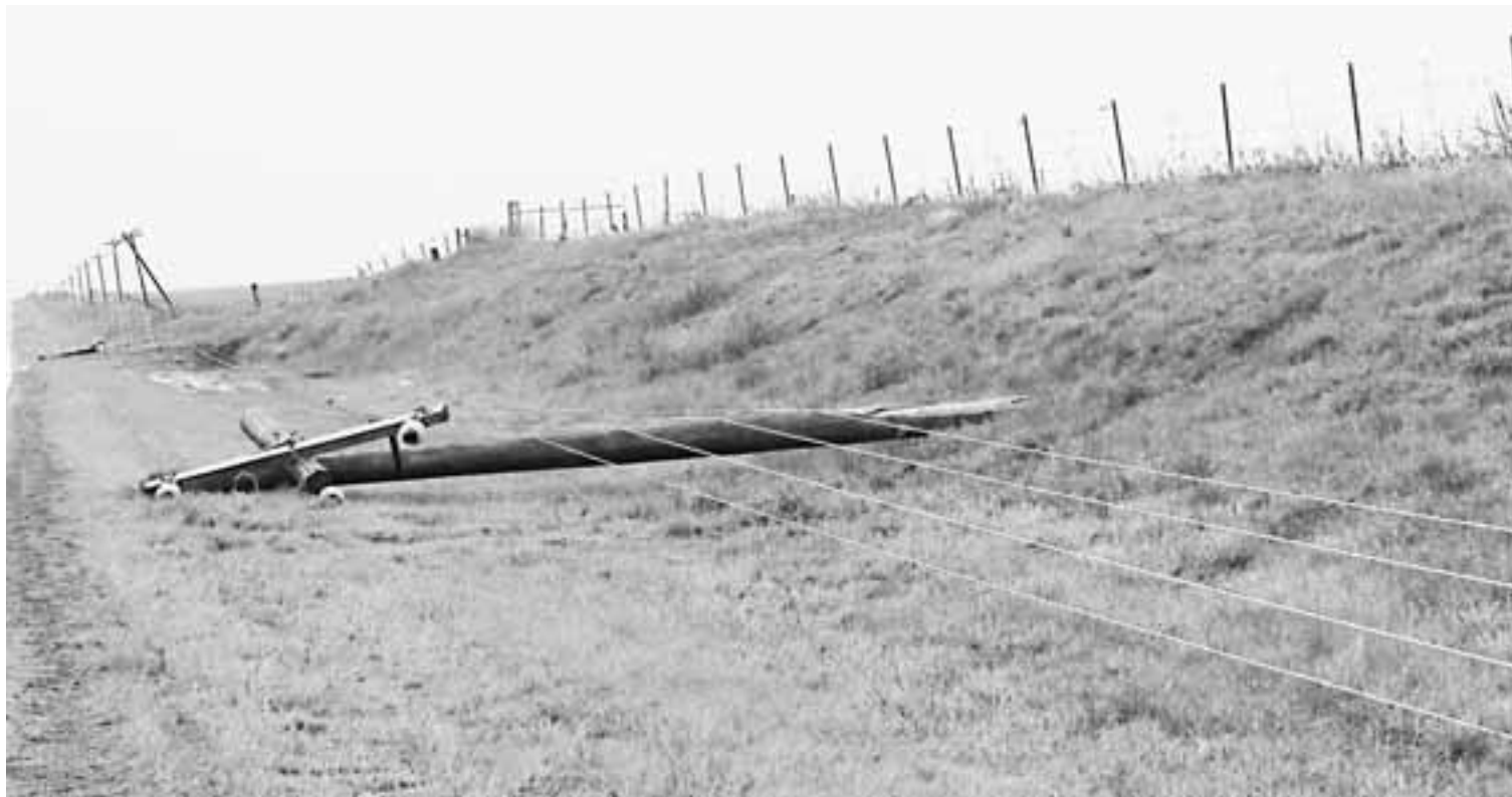
Stay away from downed power lines. These poles north of the Walters substation were damaged during the May 2 storms that swept through Cotton Electric's service territory.
