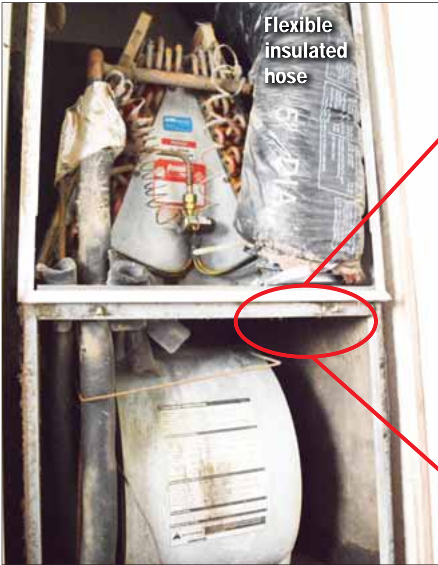
The flexible insulated hose stretches from the roof of the house down into the furnace bringing air from outside through the fresh air duct.
