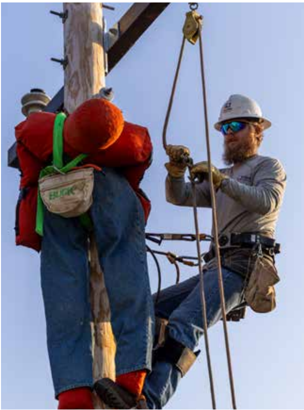
Cotton Electric Cooperative Journeyman Lineman Kyle Linthicum completes his pole-top rescue drill. Photo by Zach Young.
