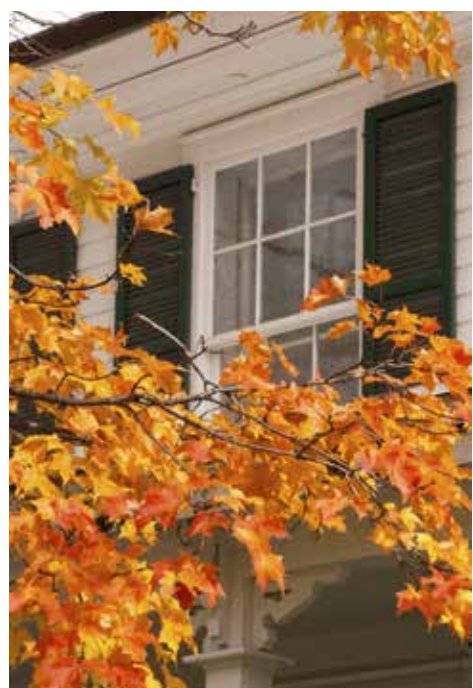
As seasons change, so should your energy efficiency habits, such as scheduling HVAC maintenance appointments and inspecting doors and windows in your home.
