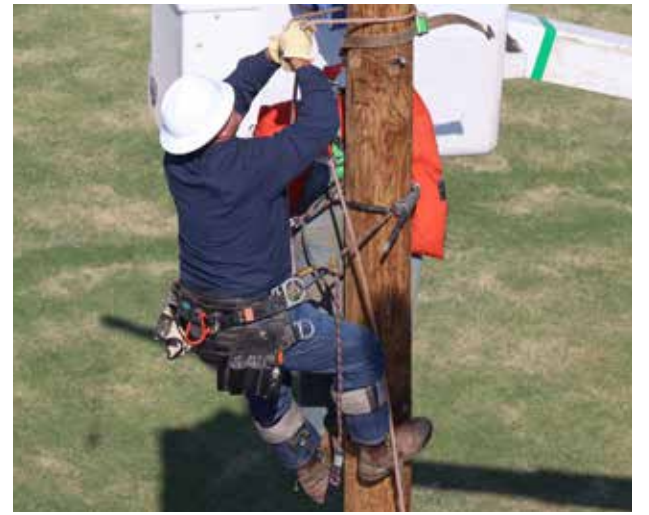
Scott Dennis, Cotton Electric journeyman lineman, performs his poletop rescue drill. Photo by Carli Eubank.
