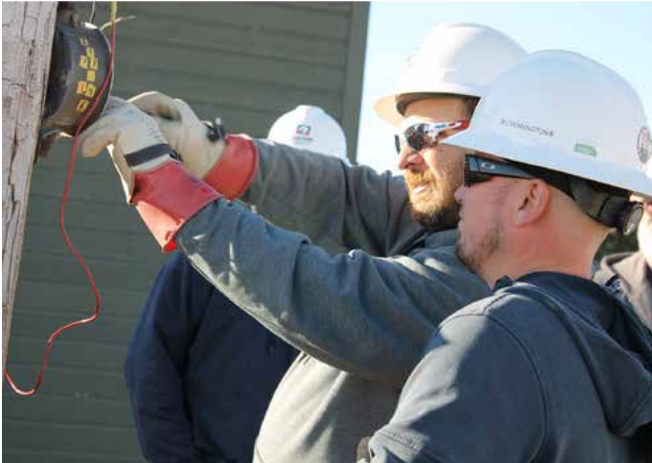
Sam Gonzalez prepares the meter base for Cody Pennington to install the final meter in a 4-year project to upgrade the Cotton Electric system.
