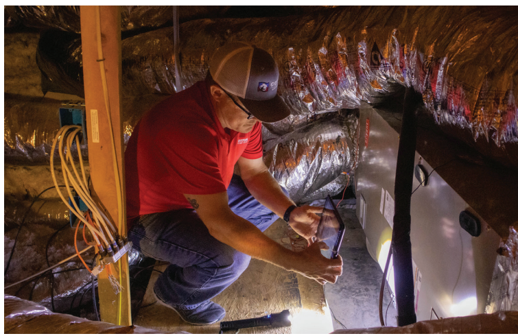
Cotton Electric Energy Efficiency Coordinator Heath Morgan checks attic insulation and efficiency. Photo by Carli Eubank.
