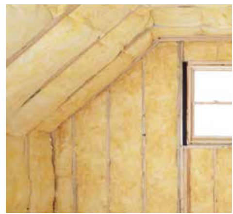
Insulated cover box and properly sealed attics are another way to avoid air leaks in your home.
