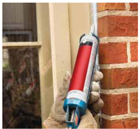
Caulking and weather stripping around doors and windows can seal air leaks and help save on energy bills.
