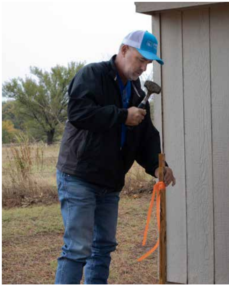
Cotton Electric Staking Technician David Break marks where lines for a new build will be laid. Photo by Carli Eubank.
